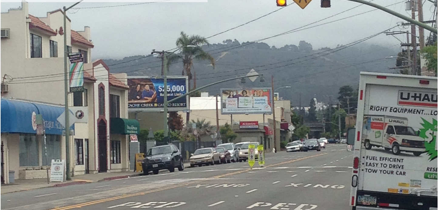
Existing Overhead Beacons and Pedestrian Paddles at one of the Mid-Block Crosswalks
