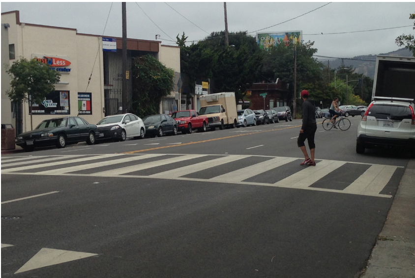
Existing Mid-Block Crosswalk Across Four-Lane Claremont Cross-Section, Existing Advanced Yield Markings
